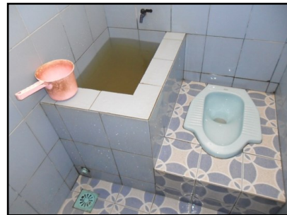
Squat toilet with water for flushing
